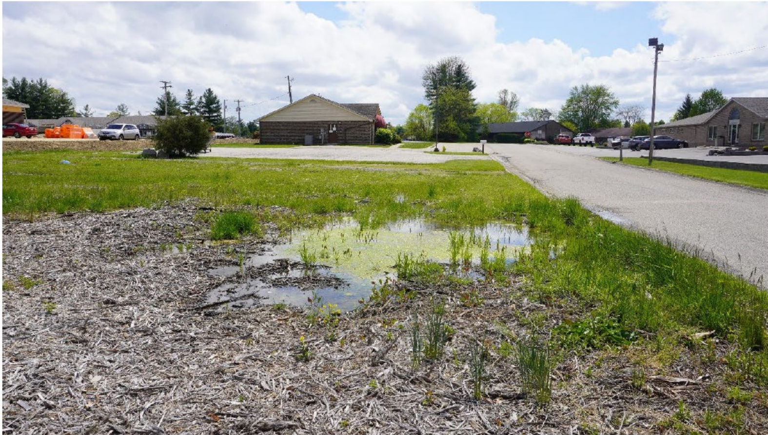
Figure 51: Ponding water located along Professional Park Dr just north of Bright Medical building (looking south towards Bright Medical building)
