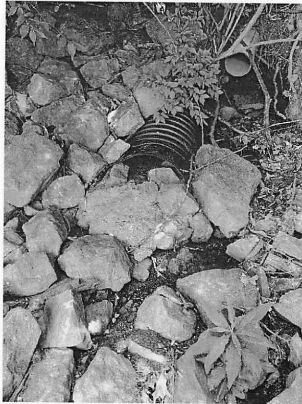
Figure 69: Obstructed stormwater outlet behind existing St. E's MOB & gutter outlet (running east to west, size unknown)
