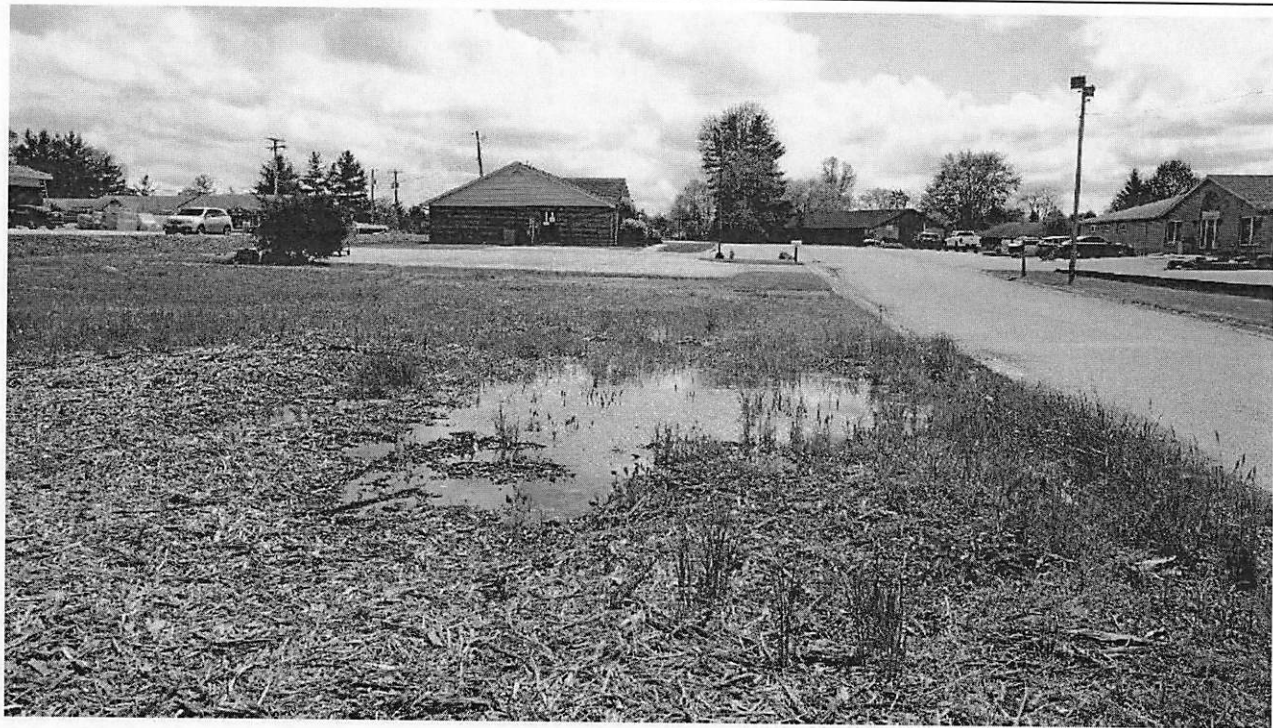
Figure 51: Ponding water located along Professional Park Dr just north of Bright Medical building (looking south towards Bright Medical building)
