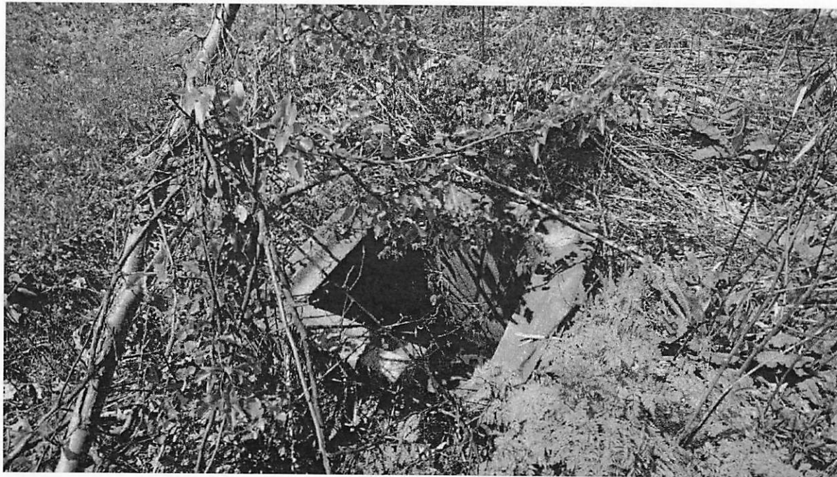
Figure 46: Top view of inlet (with no grate) located NE of the intersection of Professional Park Dr & Business Center Dr (see above)
